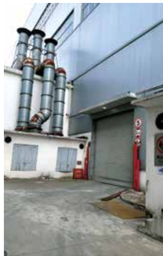
Treatment facilities of spray booth before renovation
